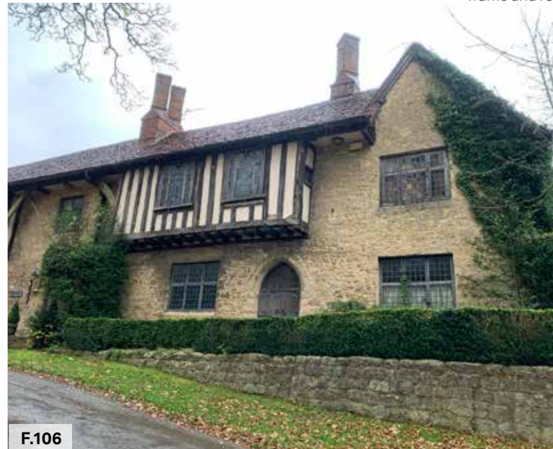
Figure 106: The mix of vernacular stone and timber frame on Old House Facade on Church Headland Lane
