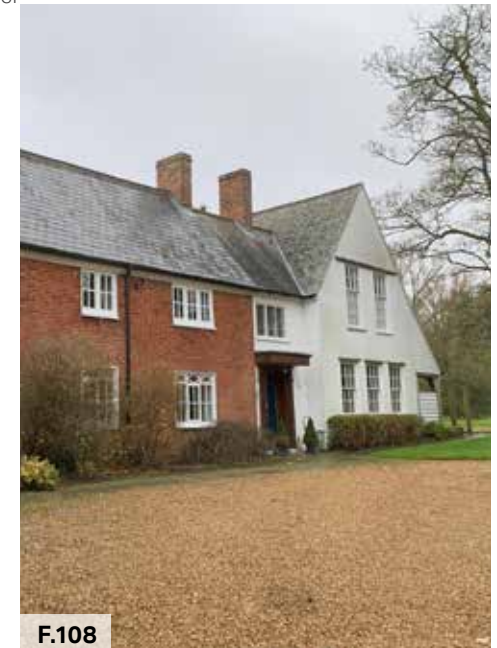
Figure 108: Mary Monk's House constructed by red brick, white render and slate roof
