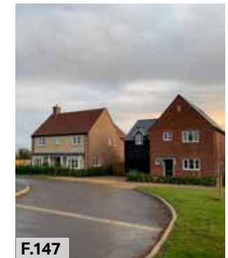
F.147 Figure 147: Unsympathetic roofline
