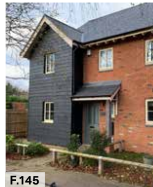
F.145 Figure 145: Full gables end at 45 degree
