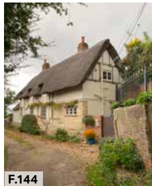
F.144 Figure 144: Full gables end at 55 degree
