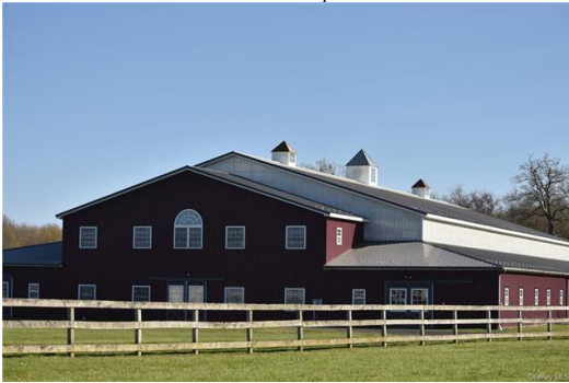
Indoor Arena/ Barn
