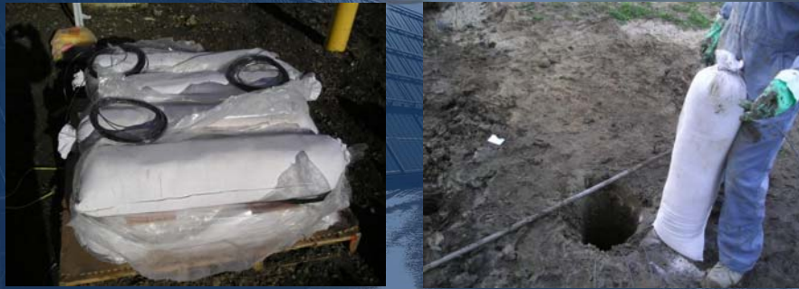
Magnesium anodes in vertical anode beds
