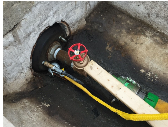
Inflatable flow-through packer
