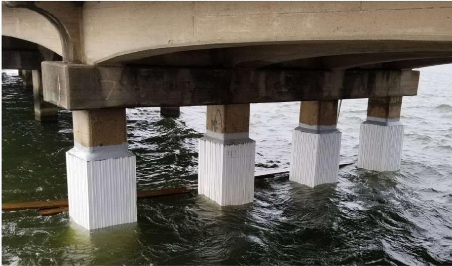
**Round PVC jacket with spacer and wiring
