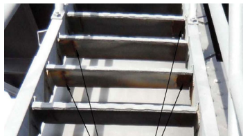
Some corrosion of steel stairs
