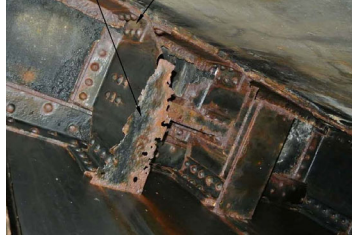
Severe corrosion of plate steel
