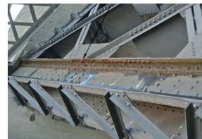
Some corrosion of superstructure elements
