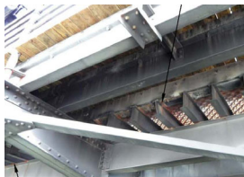
Some corrosion of steel grate support elements
