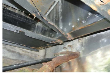
Corrosion of angle steel and return
