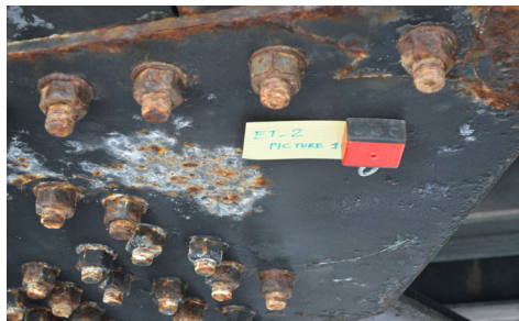
Typical Corrosion of steel plate and fasteners.
