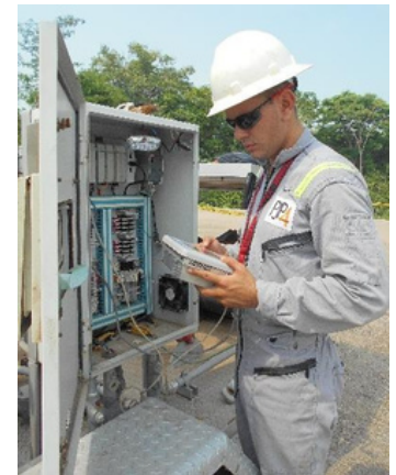
Module Inspection measurement and control
