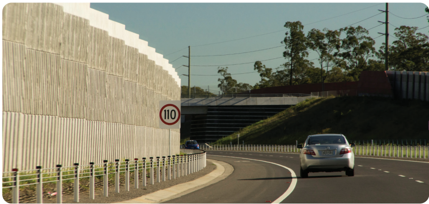
Unbroken edge line.
