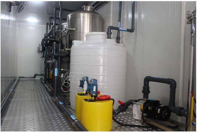
Also, some countries especially on winter time, temperature is going down. Electrical parts of containerized water treatment plant can be affected therefore we again suggest to use insulation panel with heating equipment inside of container to solve this issue.
