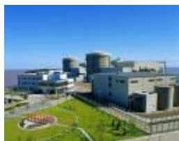
Qinshan Nuclear Power Plant
