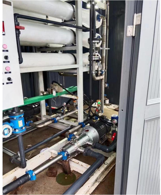
Seawater desalination ( Energy recovery booster pump )
