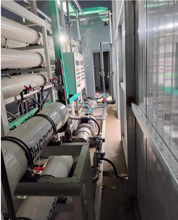
Seawater desalination ( Energy recovery booster pump )
