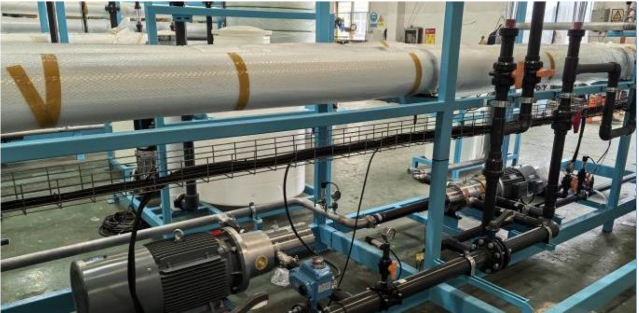
Seawater desalination ( Energy recovery booster pump )
