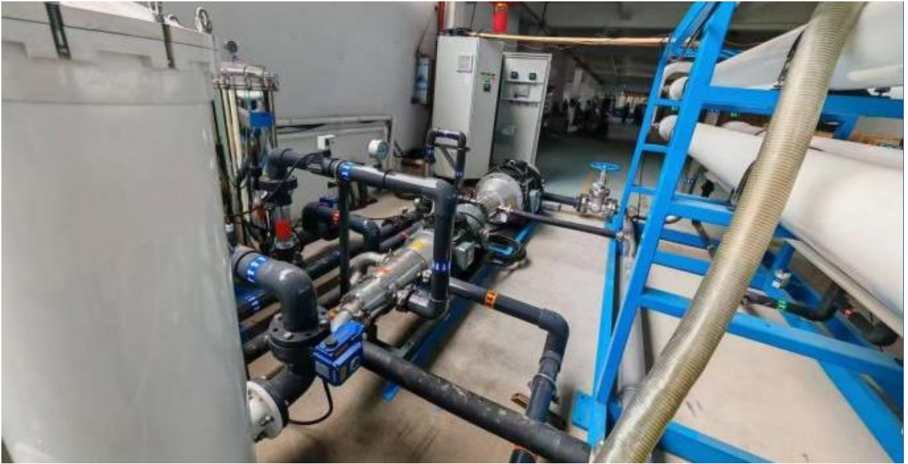
Seawater desalination ( Energy recovery booster pump )
