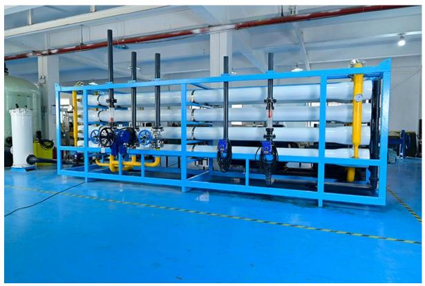
Membranes, in industrial Brackish Water Desalination Plant, are most important part. They block if parts size bigger than 0.001µm and molecular weight up to 150-250Dalton. It consists of impurities, particles, sugars, proteins, bacteria, dyes, organic and inorganic solids.
