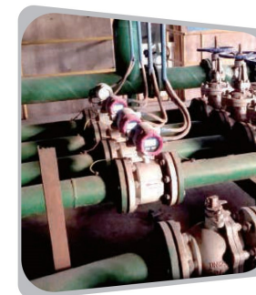
Electromagnetic flowmeter
