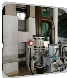
Electromagnetic flowmeter
