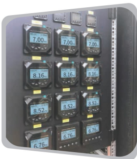
pH controller EC controller
