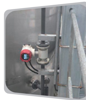
Electromagnetic flowmeter
