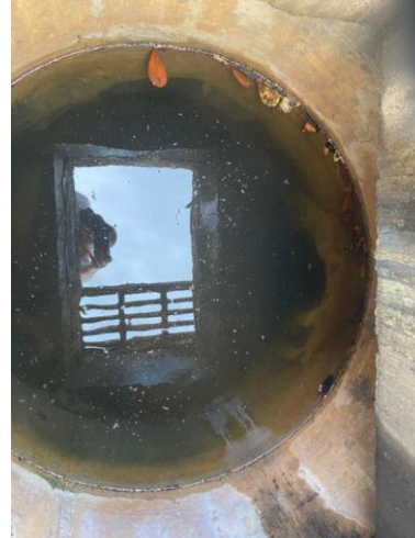
Interior of Catch Basin #1
