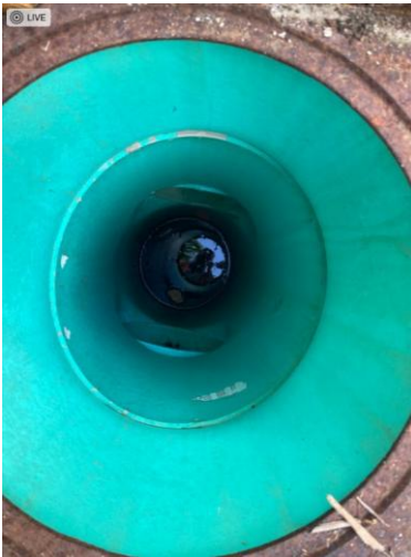
Interior of Yard Drain #2
