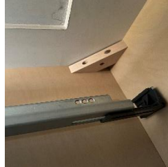
Corner Stabilizing Blocks
