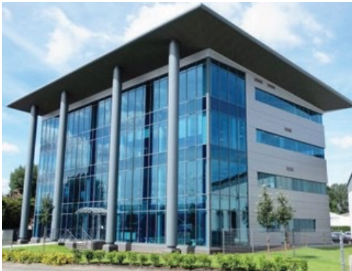
Curtain walls ( stick system) with ACP cladding
