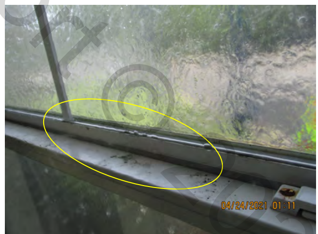
Water Infiltration witnessed at interlock Glazing Style – unit 917 – spec 2
