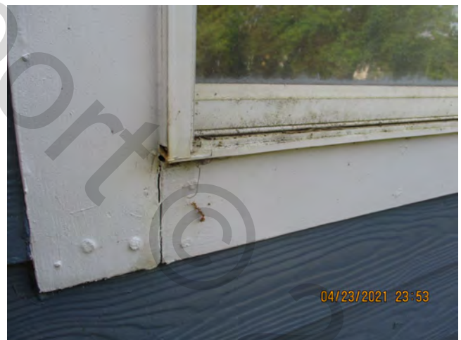
Sources of Water Penetration Identified – Unit 917
