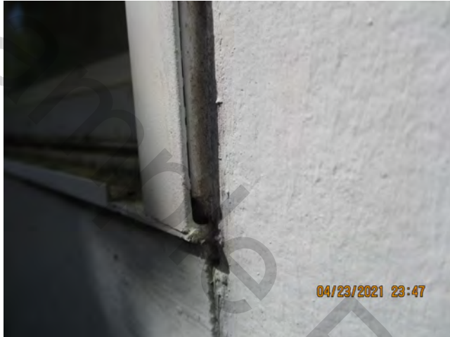
Sources of Water Penetration Identified – Unit 917
