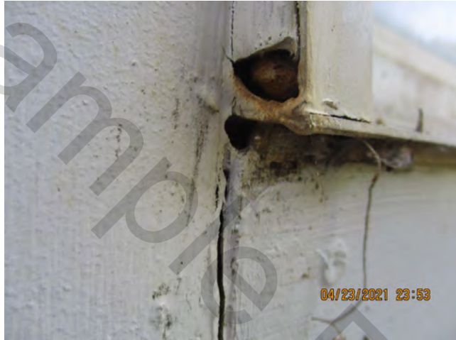
Sources of Water Penetration Identified – Unit 917
