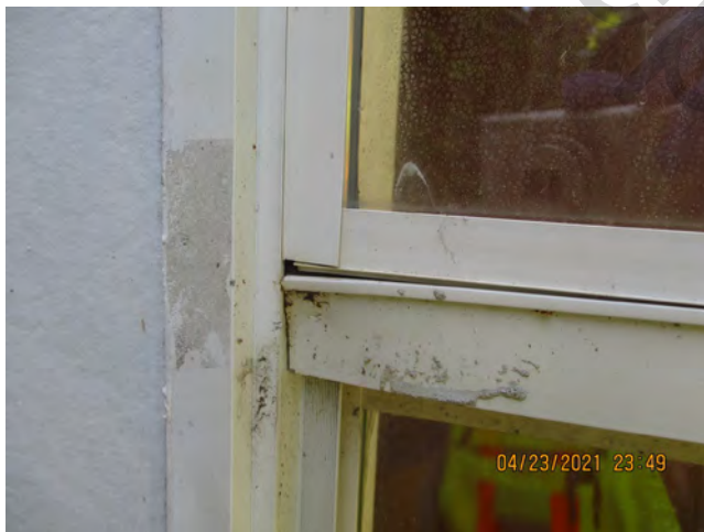
Sources of Water Penetration Identified – Unit 917
