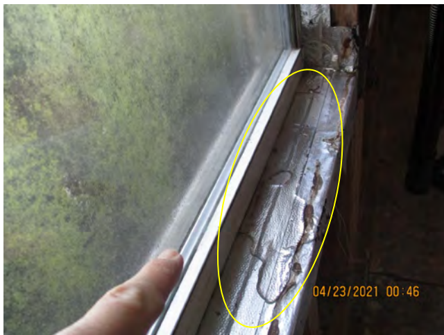
Water Penetration witnessed at window sill – unit 216 – “untested system adjacent to spec 2”
