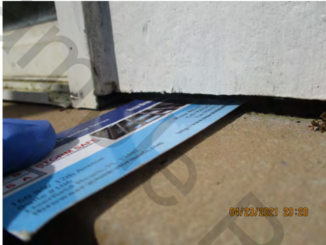
Sources of Water Penetration Identified – Unit 917
