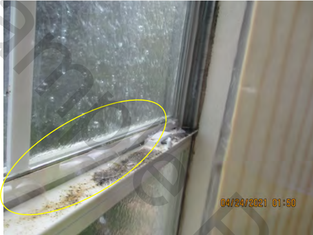
Water Infiltration witnessed at Interlocking window frame member – unit 917 – spec 3
