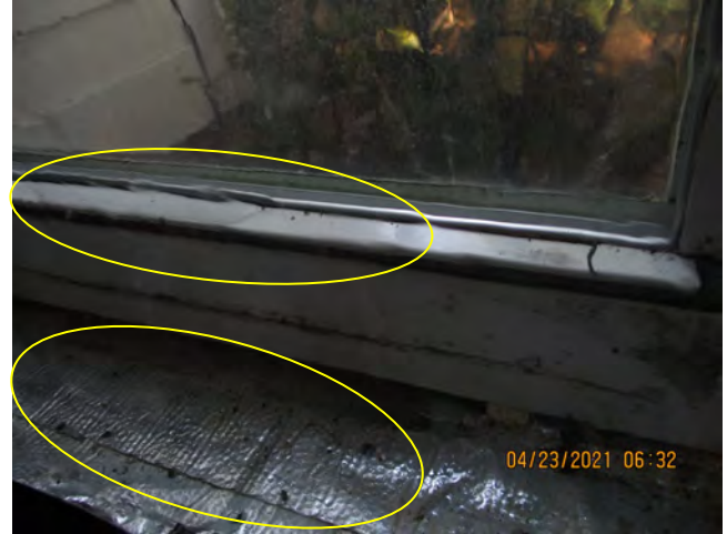
Water Penetration witnessed at window sill – unit 311 – spec 2
