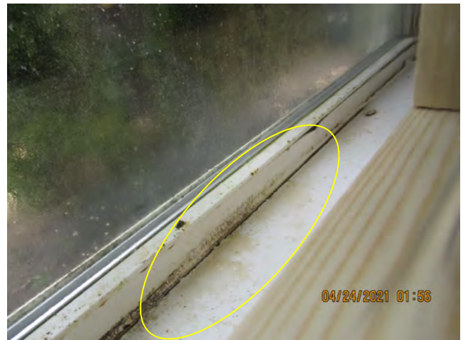
Water Penetration witnessed under the window sill – unit 917 – spec 3
