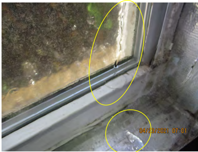
Water Penetration witnessed at interlock and sill – unit 311 – spec 3
