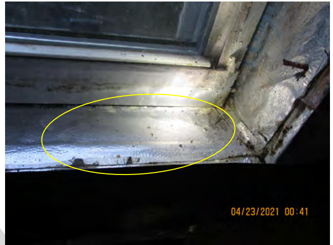
Water Penetration witnessed at window sill – unit 216 – spec 2
