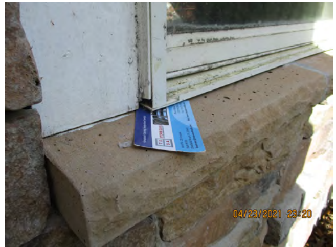
Sources of Water Penetration Identified – Unit 917
