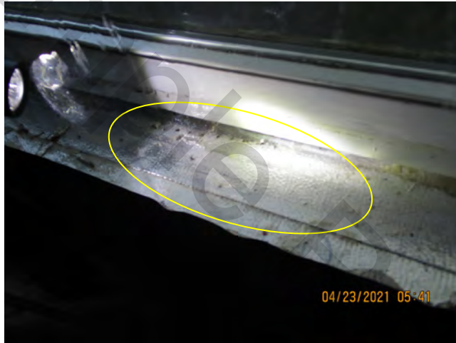
Water Penetration witnessed at window sill – unit 311 – spec 1
