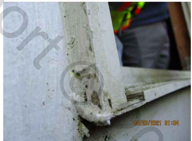
Sources of Water Penetration Identified – Unit 216
