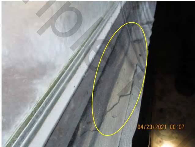
Water Penetration witnessed at window sill – unit 216 – spec 1
