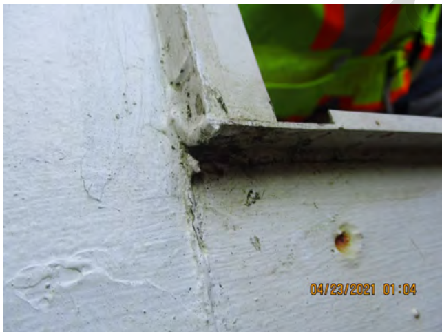
Sources of Water Penetration Identified – Unit 216
