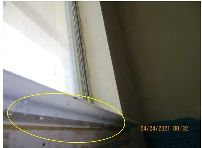
Water Penetration witnessed under the window sill – unit 917 – spec 1
