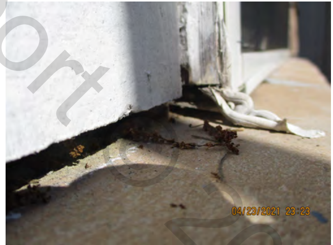
Sources of Water Penetration Identified – Unit 917
