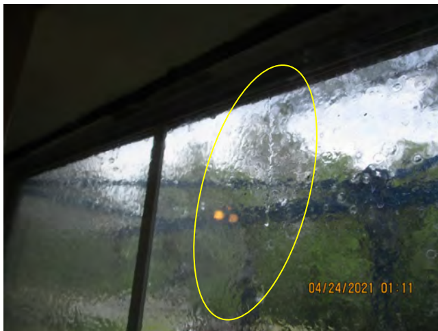
Water Infiltration witnessed at head Glazing Style – unit 917 – spec 2
