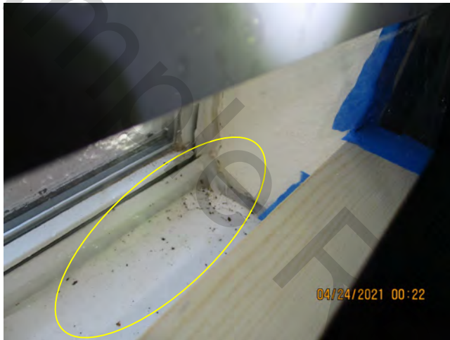
Water Penetration witnessed at window sill – unit 917 – spec 1
