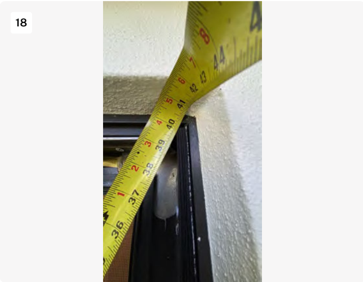
Window is installed out of square
