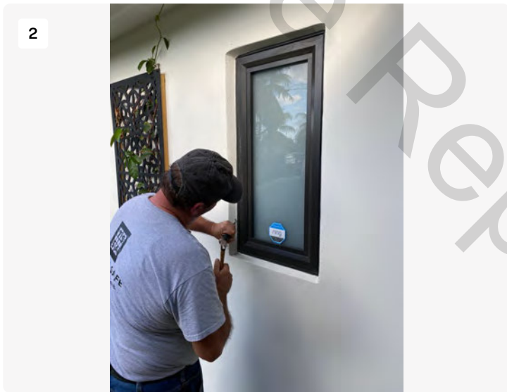
Removing exterior Stucco Reveal to inspect window installation
