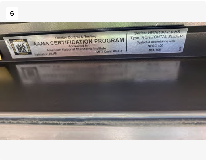
Manufacturer Sticker identifying system design pressure, thermal properties
