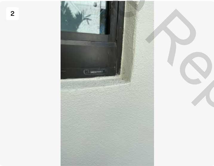
Weeping system was rendered un-functional from the interior of the sill track with Cementous material
