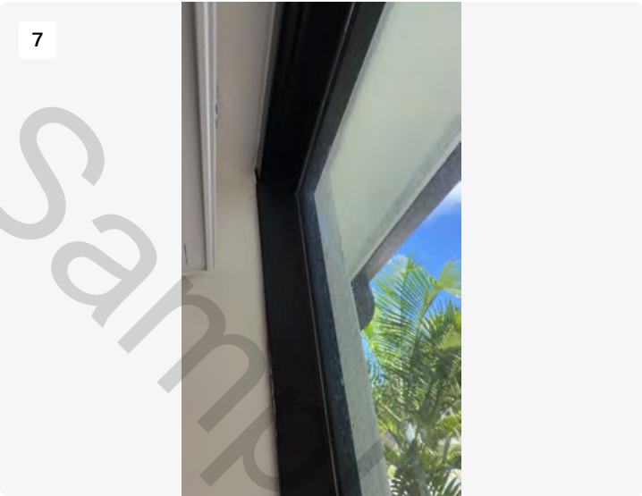
System Framed engulfed by Plaster reveal
