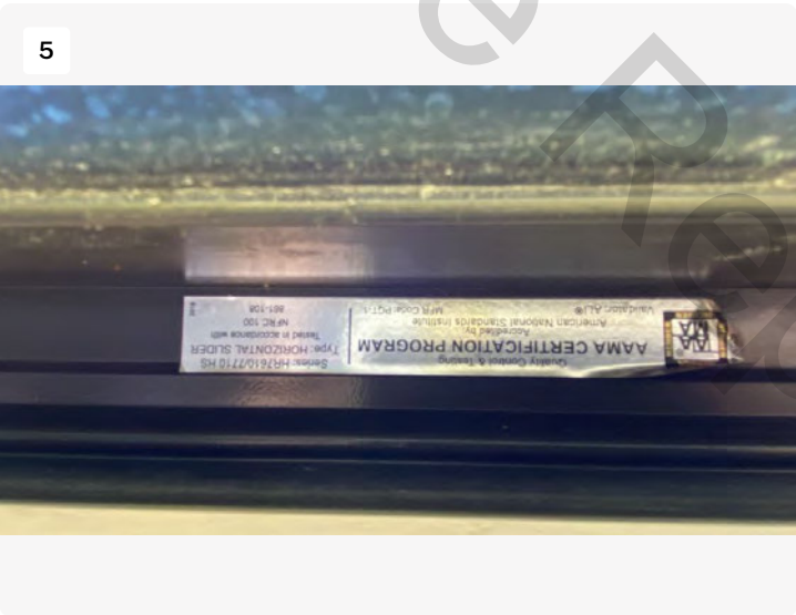
AAMA Certification Sticker showing System Manufacturer and Series and Specification
