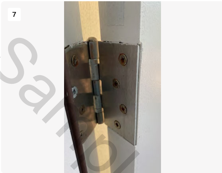
Hinge Fastener cluster installed correctly
