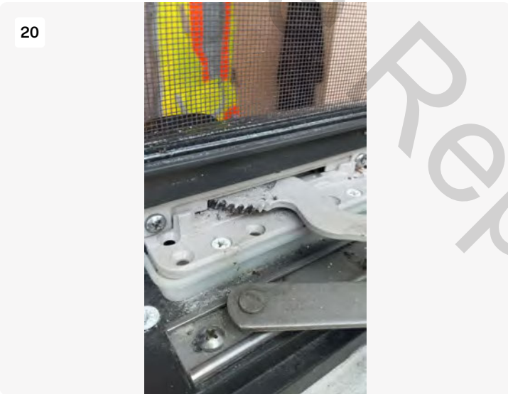
Inspecting Casement Split Arm operator and casement hinge for proper operation
