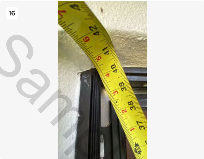
Window is installed out of square
