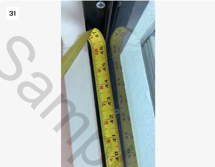
Measuring to check for header bowing
