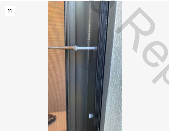
Re-installing Fastener after inspection
