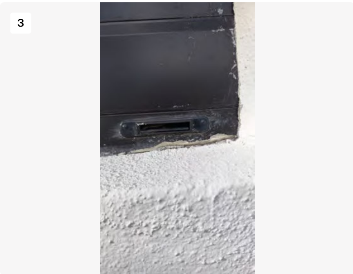
Weeping System is clean and open from Exterior
