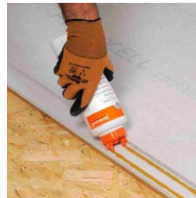
Applying FERMACELL Floor Glue to the shiplap joint
