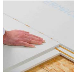
Bonding the elements with joints completely filled with Floor Glue
