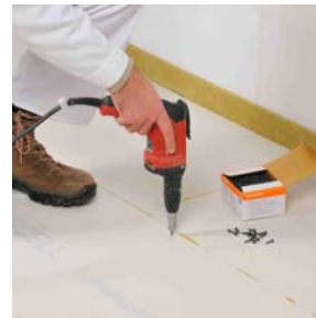
Fixing the Dry Flooring Elements with screws...
