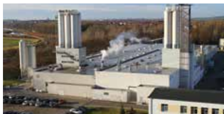
Calbe Factory, Germany
