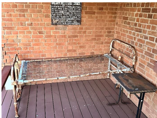
Verandah Wing, Old Thargomindah Hospital (1888)
