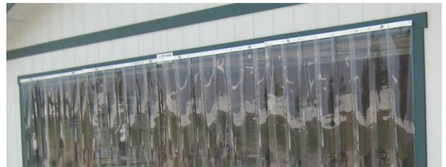
Finish installation of all panels
