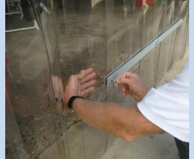
1. Locate pair of pre-perforated holes in two center slats of a 50" PARTAY Panel. Push Weight piece, with protruding studs, center stud, thru the two holes with the stud **facing away from the garage door.** Place the Weight piece with holes only, center hole, over the center stud and loosely secure a wing nut on the center stud.
