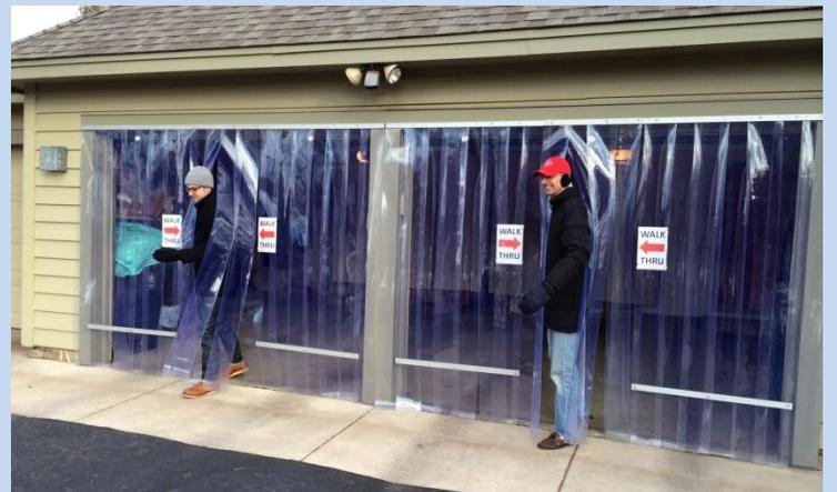
9, 10, and 18 foot wide doors utilize a narrow 26" wide panel. This small panel has minimal wind losses so weights for such are special order only. Wind Weights assemble as per above with the 26" panel in between. Now passage can be made with little motion of the wind weights.
