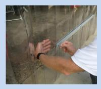
3. Arrange the slats in a balanced way so the overlaps are uniform and the panel drapes in a smooth fashion. Next secure the wing nuts snug in position to contain the panel as one unit.
