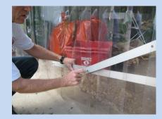
1. Locate pair of pre-perforated holes in two center slats of a 50" PARTAY Panel. Push Weight piece, with protruding studs, center stud, thru the two holes with the stud *facing away from* the garage door. Place the Weight piece with holes only, center hole, over the center stud and loosely secure a wing nut on the center stud.
