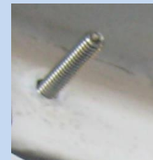
Hidden Hanger Bolt Stud Protrusion is Removable
