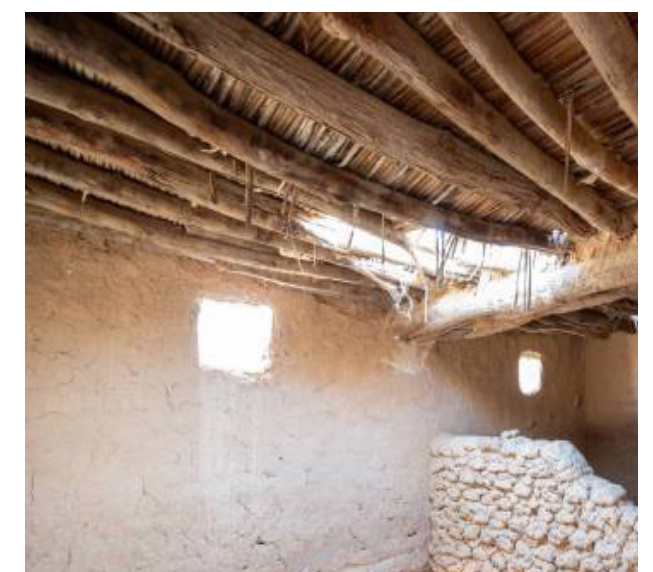
Fig. 28 Palm Leaf, Timber and Mud Roof. Charoensinphon, N. (2024).
