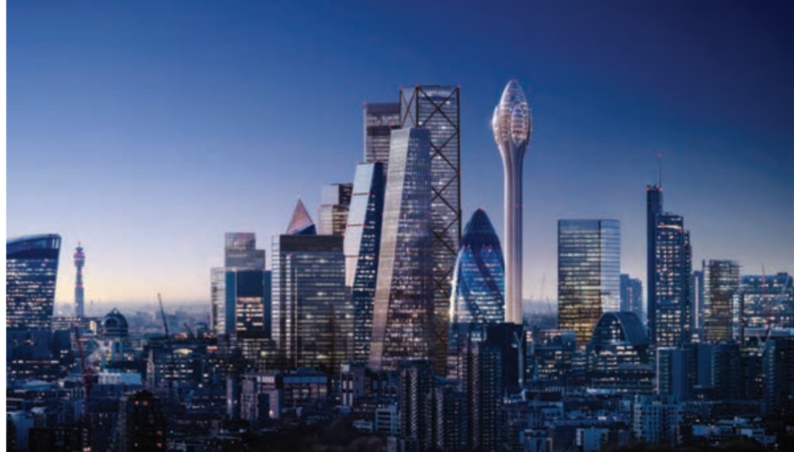
The Tulip, London, UK Client: J Safra Real Estate Architect: Foster + Partners
