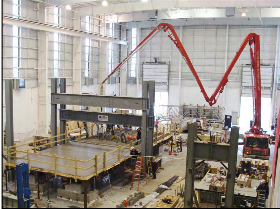
Figure 5.9: RRFC bridge concrete deck pour
