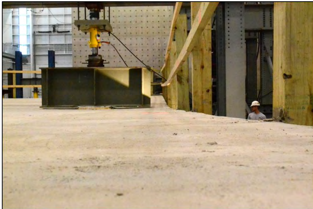
Figure 6.36: After-fracture loading of RRFC bridge (deck view)
