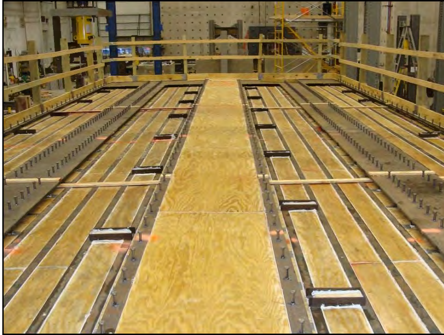
Figure 5.7: Completed formwork construction & shear stud installation
