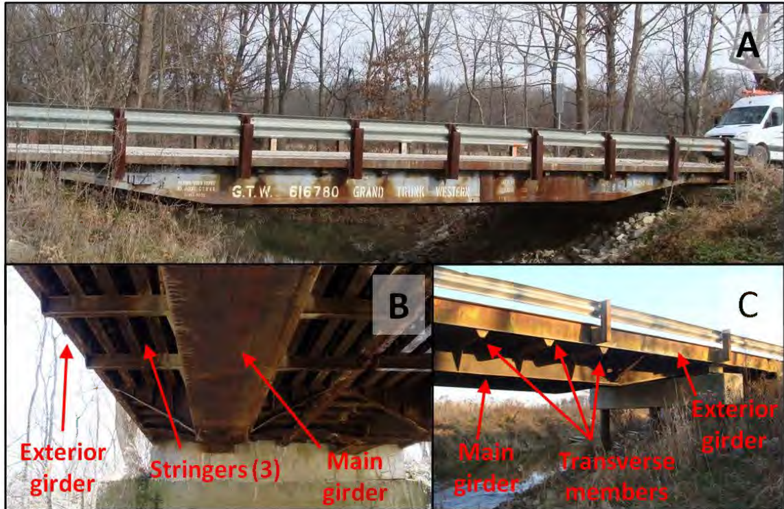
Figure 2.1: Elevation view (A), longitudinal members (B), & transverse members (C) of a typical RRFC (Provines et al., 2011)
