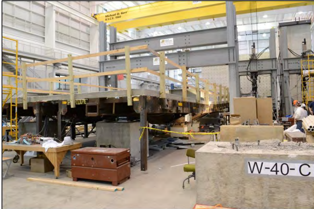
Figure 6.35: After-fracture loading of RRFC bridge
