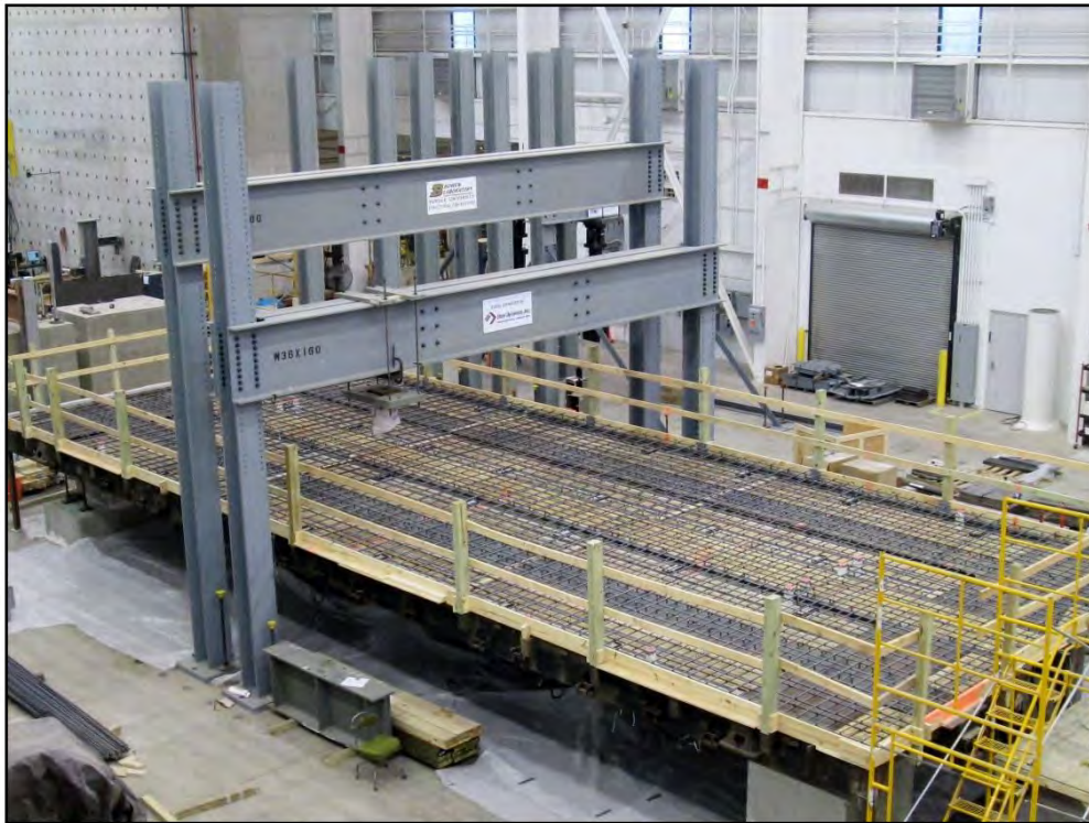
Figure 5.8: RRFC bridge after installing steel reinforcement
