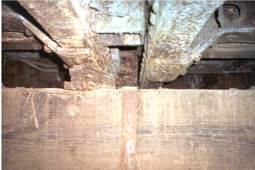
Figure 3.11. Transverse abutment support locations differed between the east and west flatcars (see Figure 3.10).
