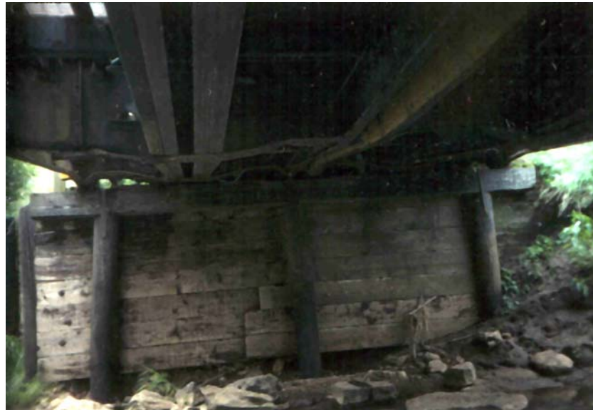
Figure 3.4. South abutment and underside of TCB superstructure.
