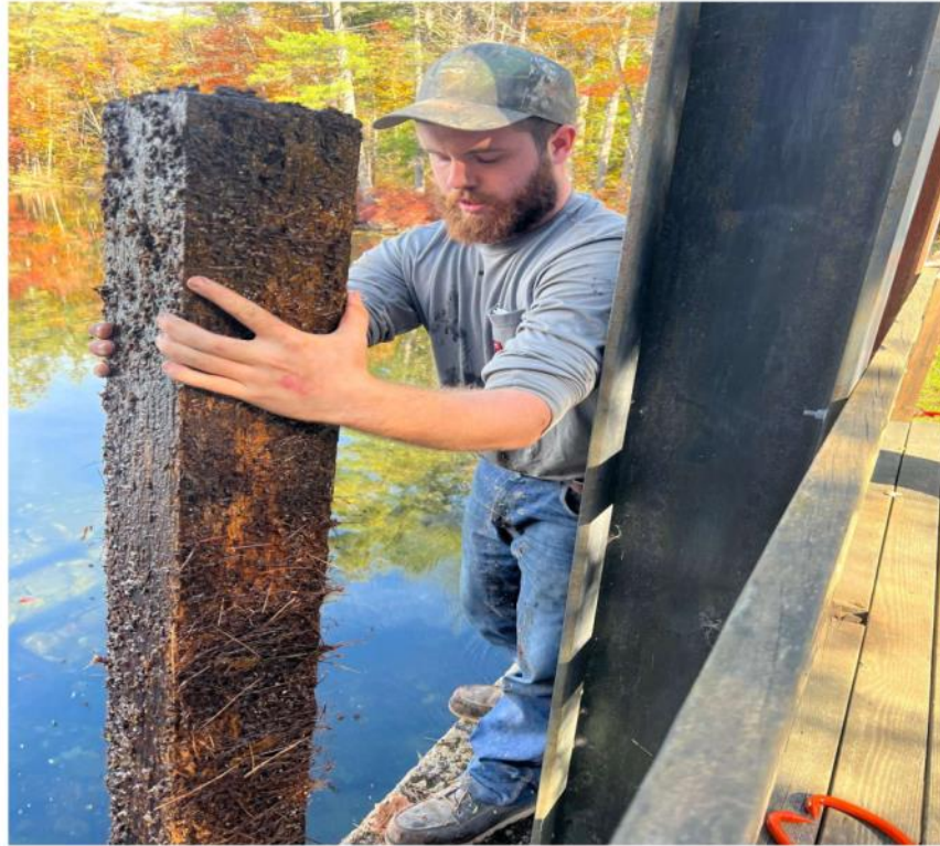
October 20th, Volunteer Holden Scott carrying water level retention board out of Colcord Pond Dam
