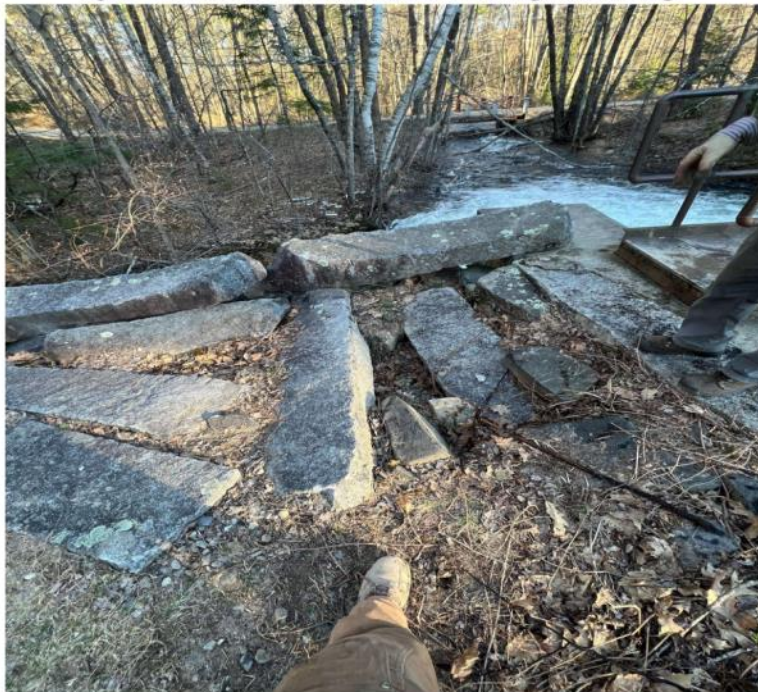
April 24th Bickford Pond, east side retaining wall sinking
