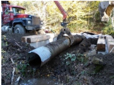
Removal of existing culvert
