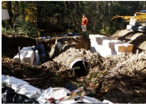
Existing culvert conveys water during construction
