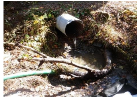
Dirty water pumped from work site
