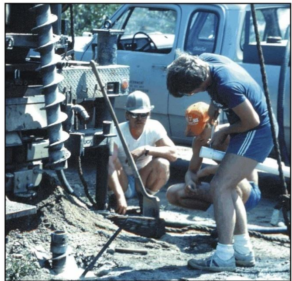
Installing a monitoring well, Washington County, Maine.
