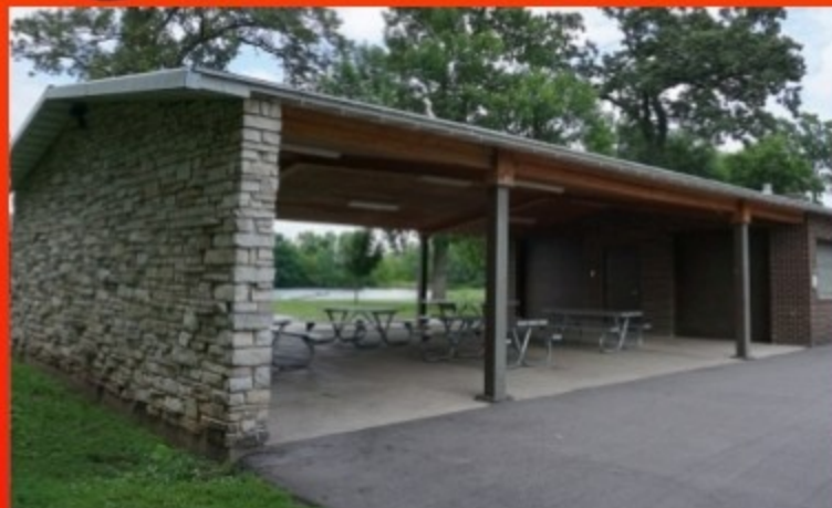
Menominee Park Shelter 1
