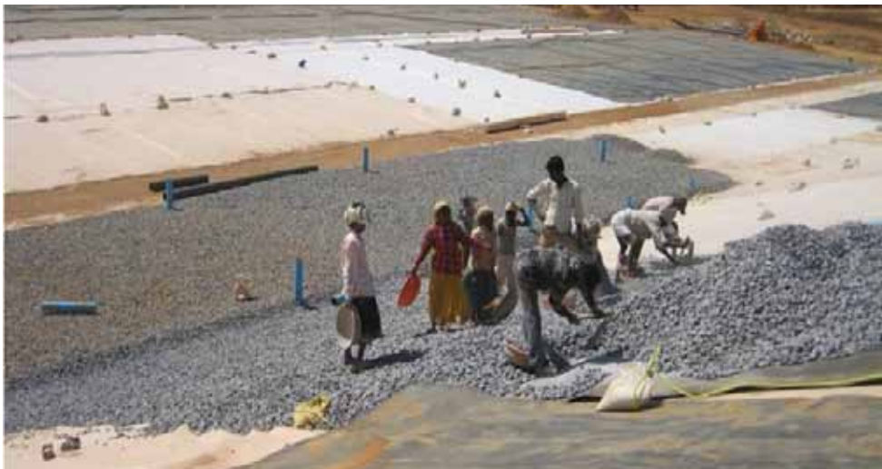
Figure 4.13: Sanitary Landfill under Construction 17
