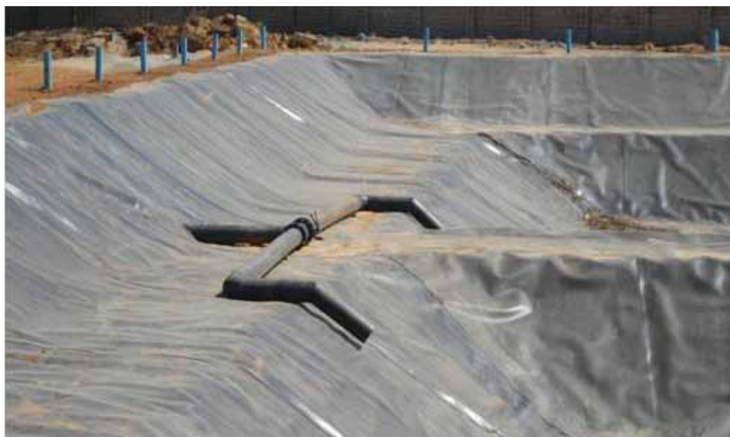
Figure 4.10: Sealed Leachate Pond with Two Basins 14
