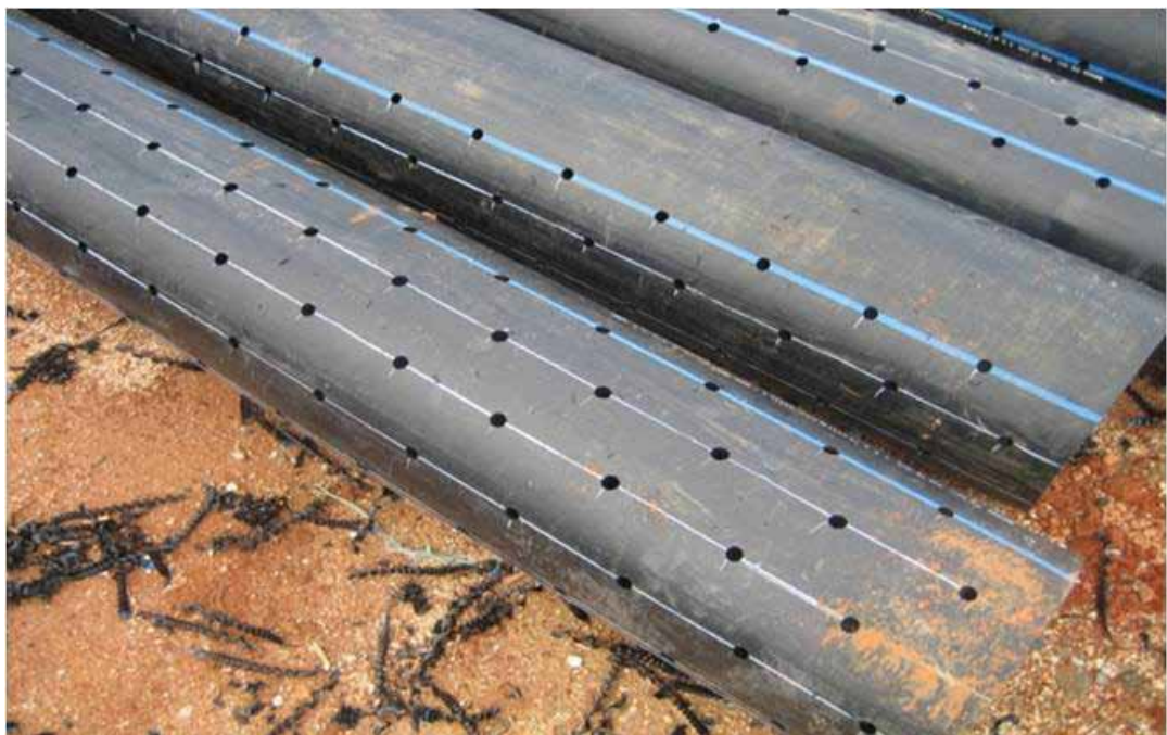
Figure 4.18: Welding of Leachate Pipes 23
