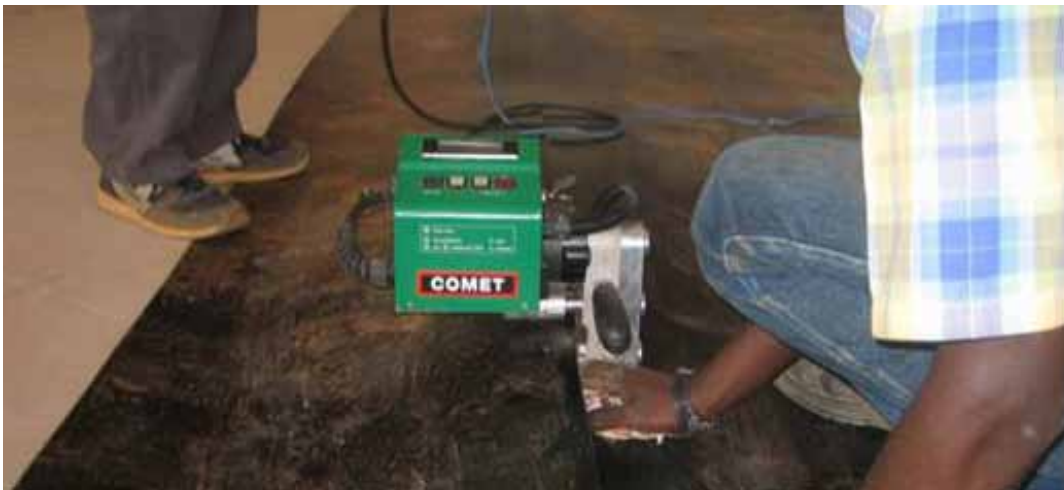
Figure 4.17: Proof of welding seams 21
