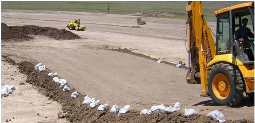
Figure 4.14: Construction of Test Field 18
