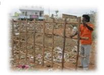
Thus each frame can accept about 400 kg waste daily. Start a second or third frame for extra 'wet' waste, do not overload in thicker layers. Build up the stack till 2.5 meter height or so, then leave for 1-3 months before giving or selling it to farmers. Do not try for a high price, try to make space on the stack frames for fresh waste. A plastic sheet covering the top may be needed only in coastal and high-rainfall areas.
