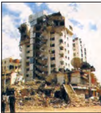
Fig. 3.3a: Destruction caused by an Earthquake in Gujarat
