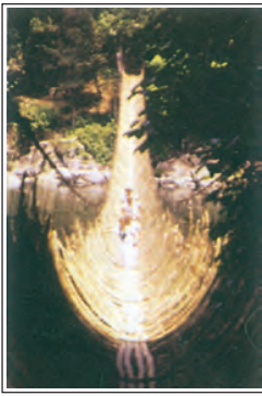
Figure 6.7 : Rope Bridge (Arunachal Pradesh)
