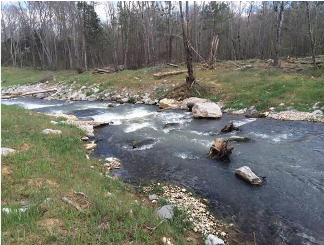
Figure 5. Boulder and Logs in a Constructed Riffle
