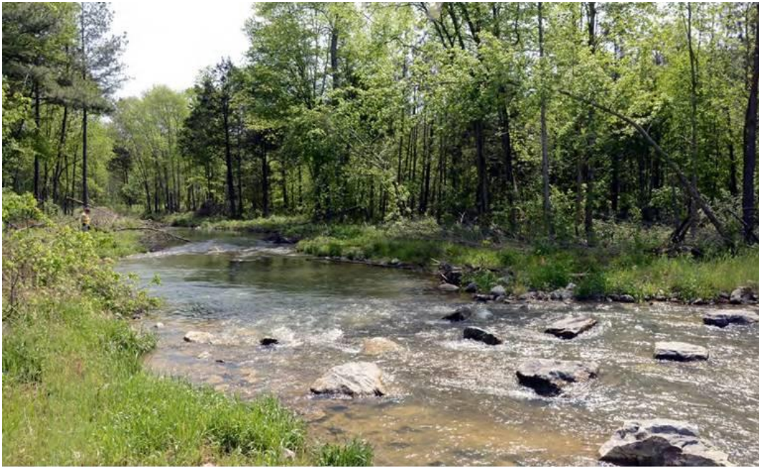
Figure 4. Boulder Clusters in a Constructed Riffle
