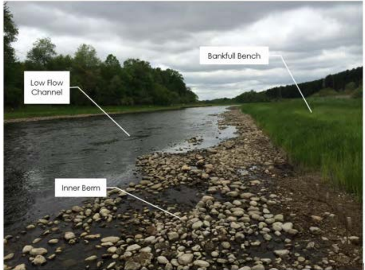
Figure 8 – Kalamazoo River – Constructed Riffle (Post-Construction)
