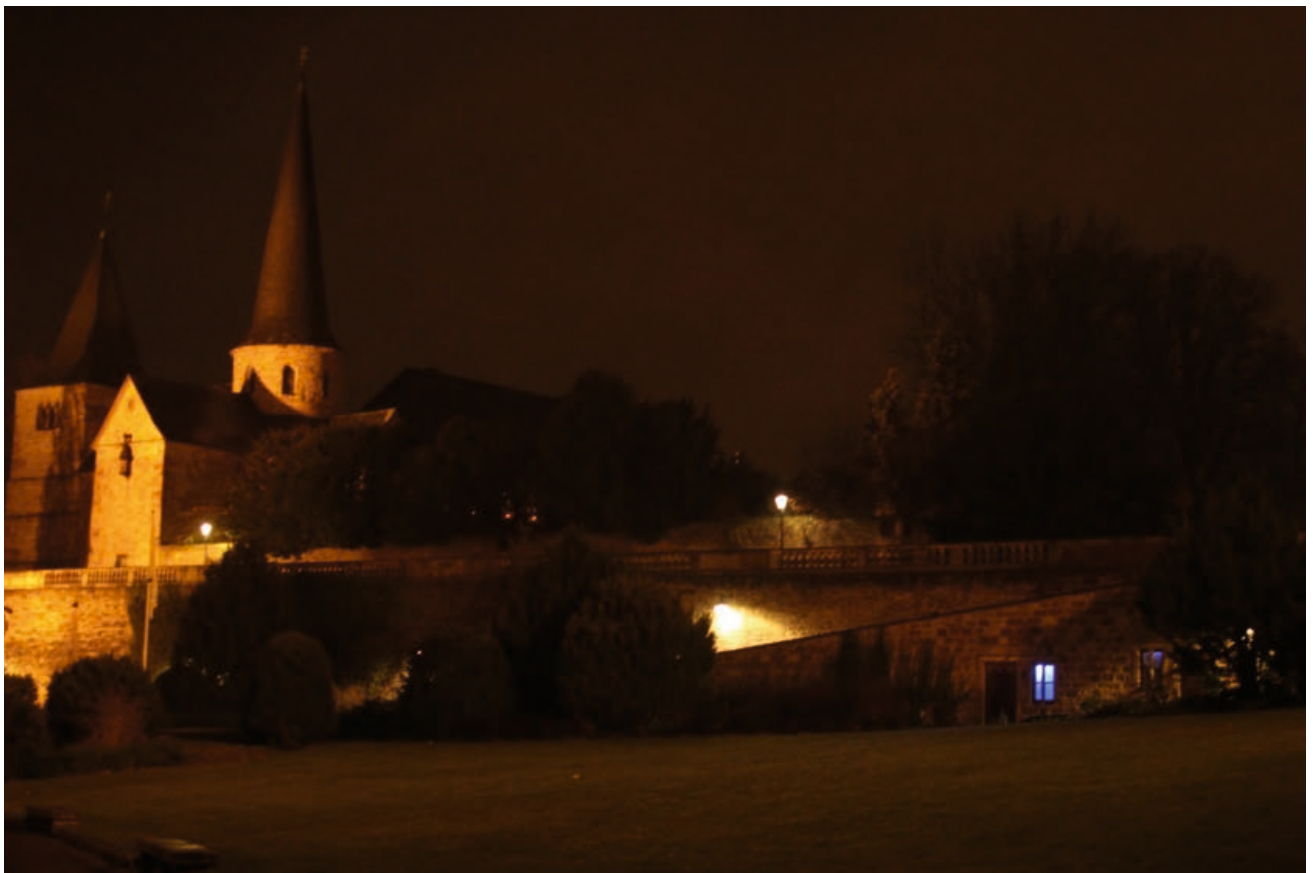
(Foto: S. Frank – retrofitted lanterns at the wall of the St.)
