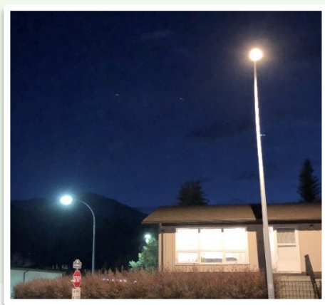
A lack of shielding causes light trespass into the windows of this home
