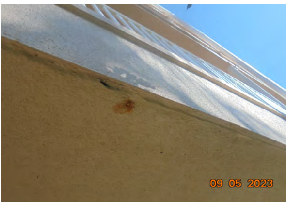
39 Delaminated Stucco
