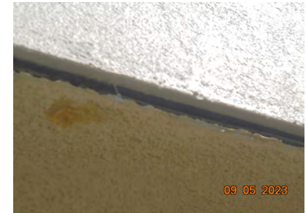
38 Delaminated Stucco
