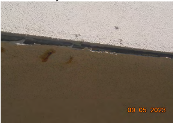
37 Delaminated Stucco
