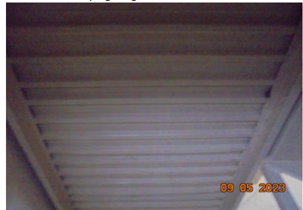
30 Metal Pan Below Landing (Stairwell)
