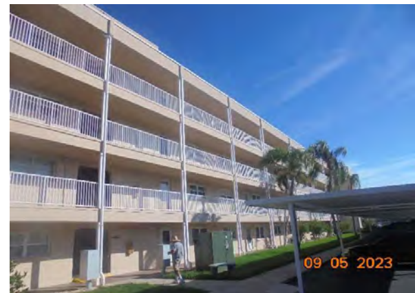
4 Left Side of Building
