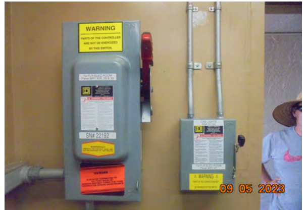
16 Elevator Disconnects
