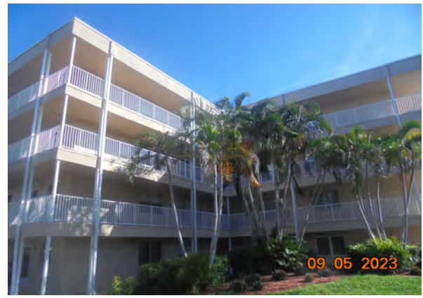
2 Right Side of Building
