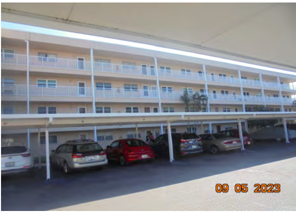
1 Front of Building
