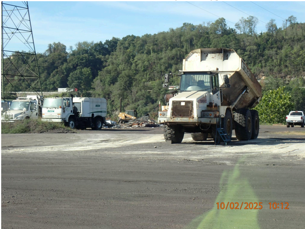
PA020318 - Track-out of gypsum sand
