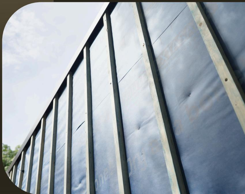
For completeness, HighLine™ battens can be used in conjunction with HighFlow™ Project battens at top and bottom of cavity to create a complete drained vented cavity system and where fasteners are required at top and bottom of the cavity for cladding systems [for accessories and flashing etc.]. This solution remains compliant with proposed condensation management requirements of NCC 2025 [climate zone 6-8].
