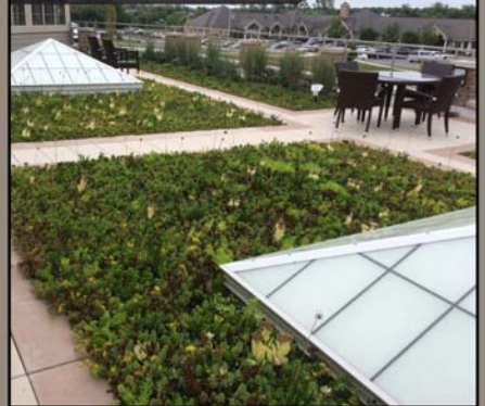
LIVE GREEN ROOF | FT. WAYNE, IN
