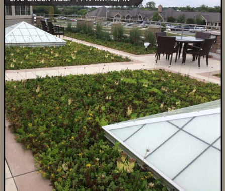
LIVE GREEN ROOF | FT. WAYNE, IN
