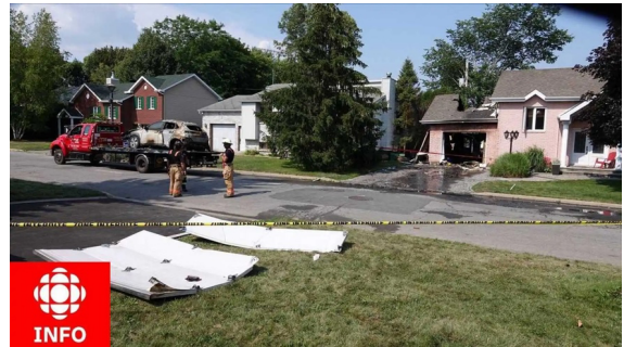
Fig. 7. Ashburn VA after explosion launched garage door across street. Failure of charging car battery filled garage with explosive hydrogen, similar to failure of BESS systems.
