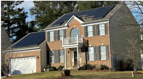
Fig. 6. Solar panels which may connect to garage BESS.
