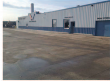
New full length truck scale & building enhancement in 2021
