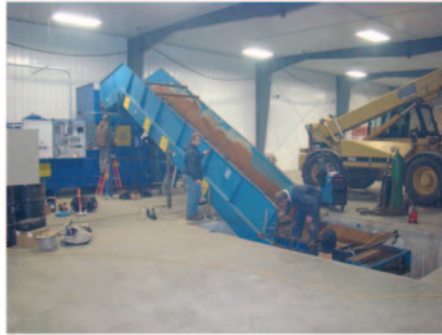
Installation of non-ferrous baler in January 2013
