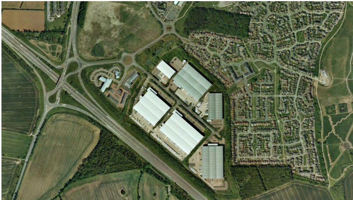
January 2009 - The addition of the last structure, making the site the same as it is today.
