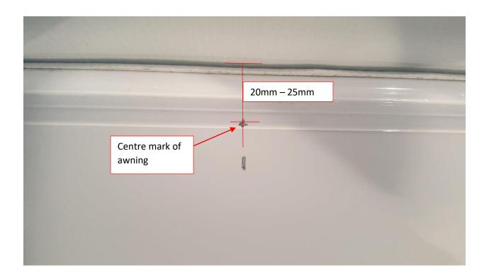
Centre the bracket with the marking at center of awning on the van and with a texta mark the required holes for the pop rivets.
