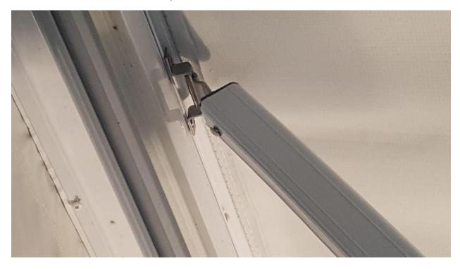
**Step 18**Extend out the front telescopic section and fit spigot into the hole in the roller. Once in place tighten the center black screw which will then hold the rafter in position.
